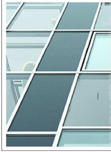
Curtain Walling To Hangar Door Satin Anodised Aluminium/ Clear Glazing With Antistatic Spandrel Lower
